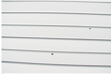
Hail damage Small
